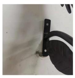
To use with wall fixings (provided) please drill two 0.5cm holes as shown.
