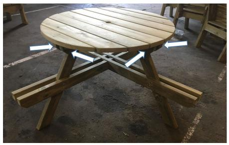
2) Next, lift the table top in place so that the legs slot between the runners underneath the table top. Once the table top is sitting straight and is fully pushed down onto the legs, screw two 4" screws through the table top runners into each of the legs, as shown by the arrows.
