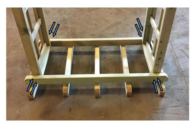
2) Fix the 4 angle braces in place with 16 x 3" screws as shown by the arrows below.
