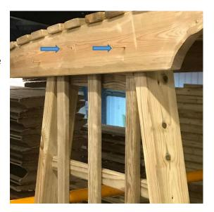
6) Next, place washers and nuts on all the bolts that you have inserted, and fully tighten, so that the swing is secure.
