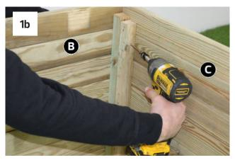
Set out Part B Back panel with Part C side panel and secure using 2x 60mm screws 1 at the top and 1 at the bottom approx. 40mm down/up from the end, ensuring all corners are square and flush as shown in Fig. 1a & 1b.
