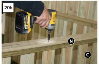
Place Handrail (N) onto Side Panel (C) and fix using 5 x 45mm Screws. Repeat procedure for remaining Handrail (N) on other Side Panel (C).
