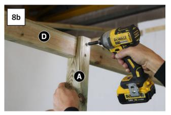
Position 1 x Bearer (D) into notches in Posts (A). Allow a 30mm overhang beyond back of rear Post (A) and to Rear Post fix using 2 x 60mm Screws. Fix Bearer (D) to front Post (A) using 2 x 60mm Screws.
