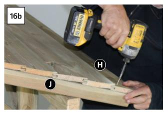
Position 1 x Roof Batten (J) beneath roof boards and fix using 4 x 45mm Screws.
