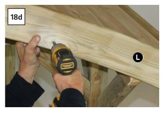
Ensuring Roof Battens (J) and all board ends are covered, attach 2 x Fascia's (L) (Ensure correct orientation of Facia) to Roof Battens (J) using 6 x 45mm Screws. (3 x Screws per Fascia (L).
