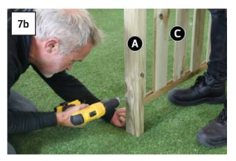
Fix remaining Posts (A) (Notch facing outwards) to Side Panels (C), at a height of 90mm from base of Post (A), using 2 x 80mm Screws.
