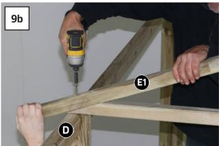
Place 1no. Truss (E1) directly above front Posts (A) and fix using 2 x 120mm Screws (1 x Screw per end)
