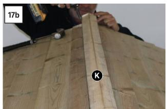
Position Roof Capping (K) at apex of roof and fix using 8 x 45mm Screws (4 x Screws per side).
