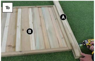
Place Back Panel (B) at a height of 90mm from base of Post (A), ensuring notch in Post (A) is facing outwards, fix in position using 2 x 100mm Screws.
