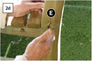
Insert 4no Cross Dowels into 10 mm holes to rear of Back Assembly (C) ensuring slots face outwards (as shown in Fig 2a, which allows for aligning dowels with bolts using a slot head screwdriver). Position the Back Assembly between side assemblies (Fig 2b) and insert 2no bolts per side and carefully thread bolts into cross dowels (Figs 2c & 2d).
