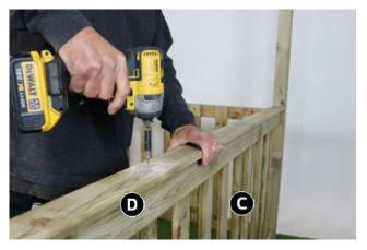
Place 1x Handrail Cover (D) onto Handrail (C) and fix using 4 x 45mm Screws. Repeat for remaining 2 x Handrail Covers (D) and Handrails (C)
