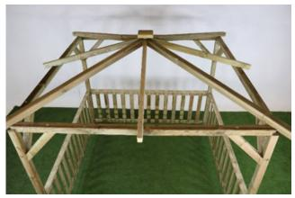
Attach 1x Centre Rafter (H) to Final Block (G) using 1x 100mm Screw and to Ring beam using 1x 100mm Screw.
