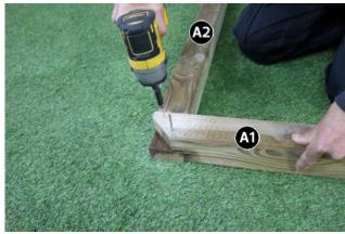
Set out Ring Beams A1 & A2 as shown above and fix in position using 8 x 60mm screws,  $2 \times 60$ mm Screws per corner.
