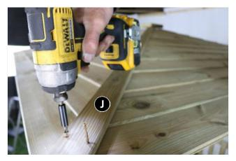
Place 1x Long Cover Strip (J) over joint in roof boards and under finial block capping (angled cut beneath capping and facing upwards). Fix in position using  $8 \times 45$ mm screws ( $2 \times 45$ mm screws per end,  $2 \times 45$ mm either side of centre).
